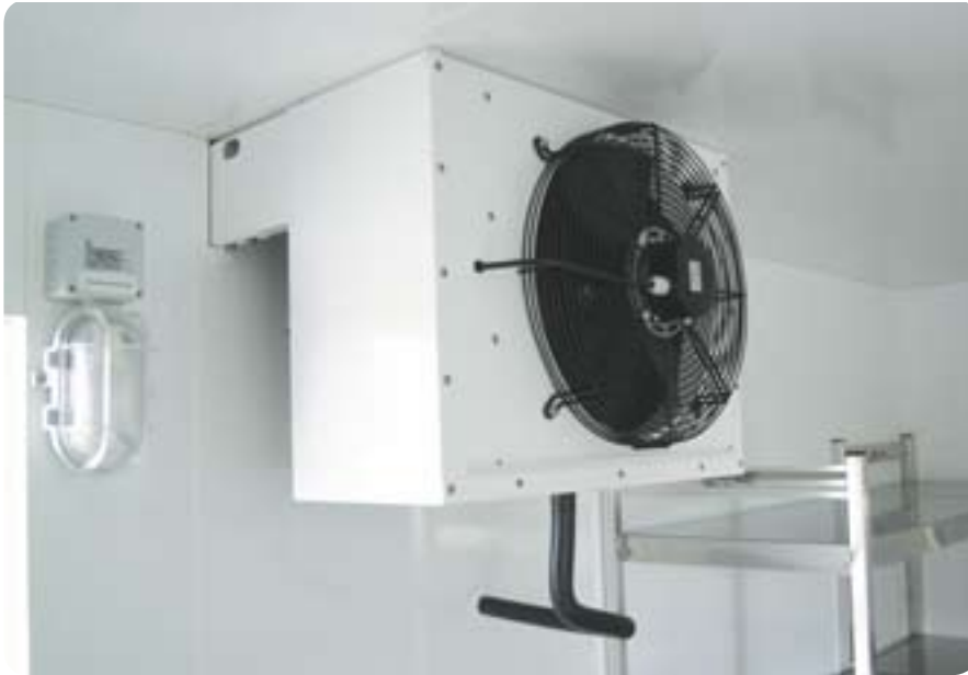
Wall-hanging unit (evaporator) installation
