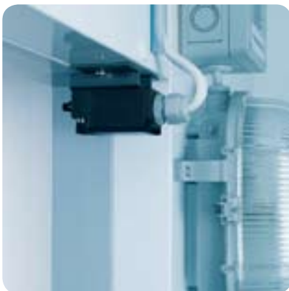
Door contact switch for automatic control
